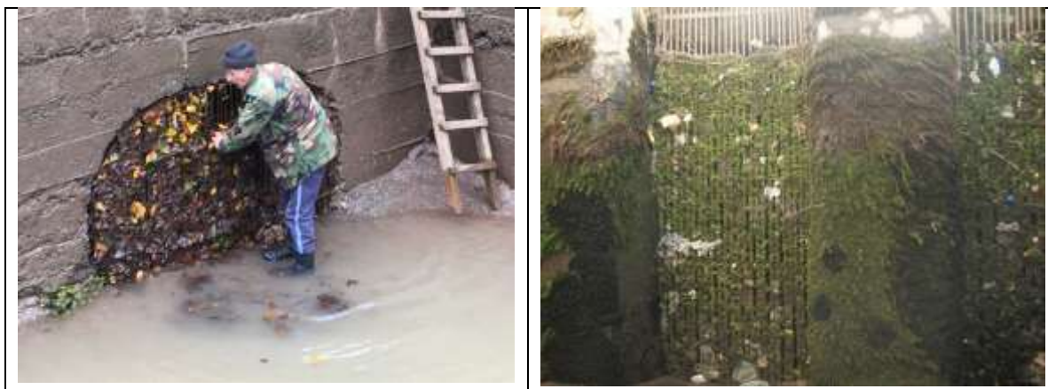
Fig. 2. Clogging of the settling tank screens. A) Fallen tree leaves in the autumn at the Chirukhi SHPP (Georgia), b) Clogging of the small screen at the Shaki SHPP (Armenia) with aquatic vegetation and debris
